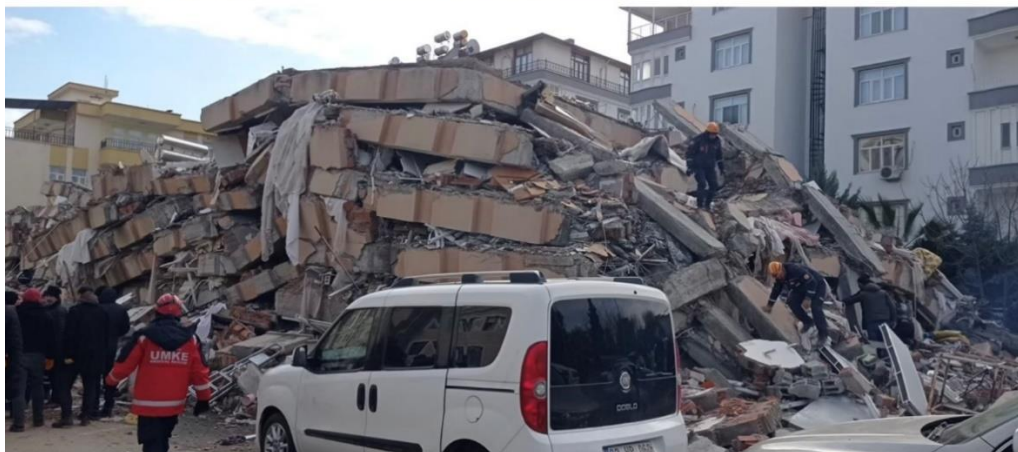
Figure 3.10: Collapsed buildings in Adiyaman city center.
