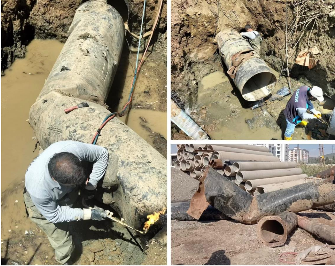
Figure 6.2: Repair process of the damaged \Phi 700 mm steel pipe.
