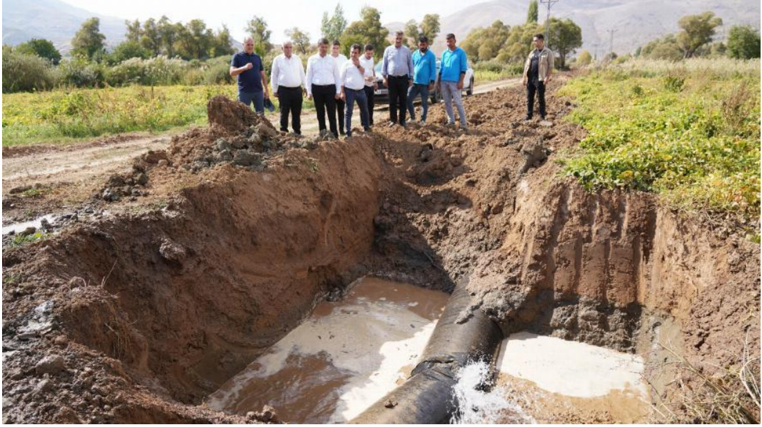
Figure 6.1: An example from field studies conducted on the Havşeri transmission line [Adıyaman Municipality, 2024].
