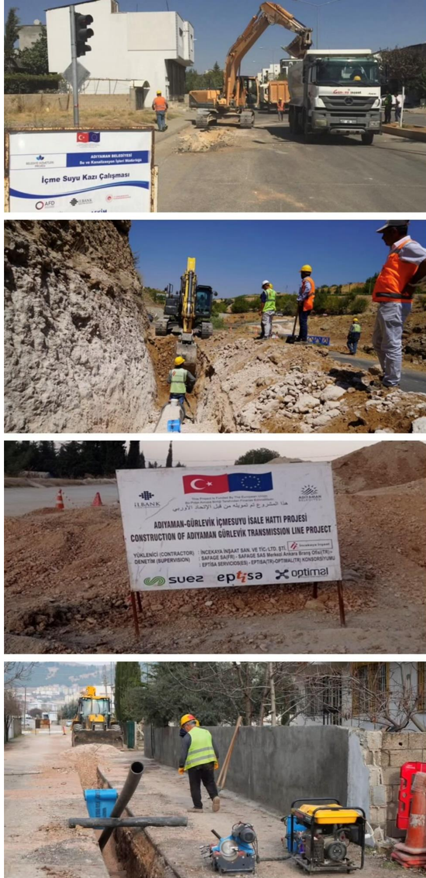
Figure 5.5: Implementation photographs of MADAD and FRIT II frameworks.
