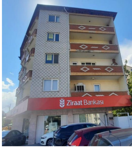
Figure 4.18: The building located in the Kümbet district of Sivas city centre.
