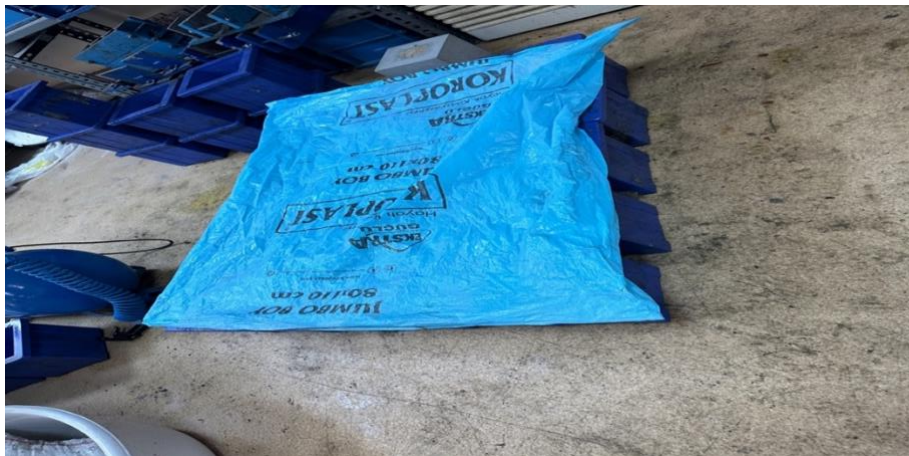
Figure 9: Covered Concrete Molds.
