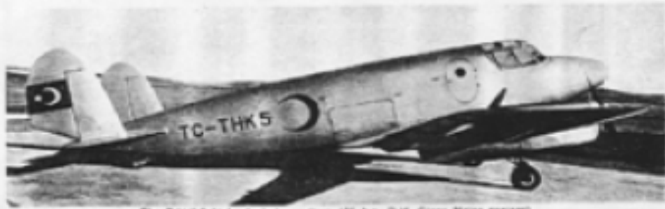
The T.H.K. 15 Light Ambulance (two 120 h.p. D.H. Gipsy Major engines).
