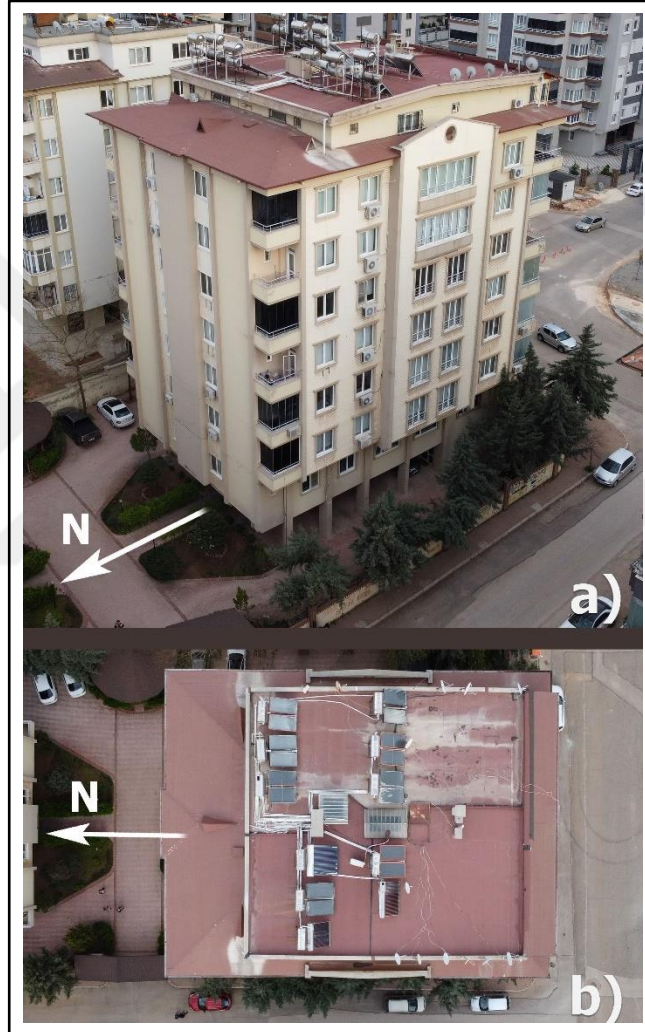
Figure 4.8: Aerial photos of the Building 2 from (a) side and (b) top.
