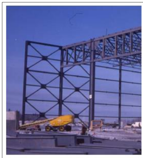
Figure 1.13: Multi-Tiered Concentrically Steel Braced Frame.
