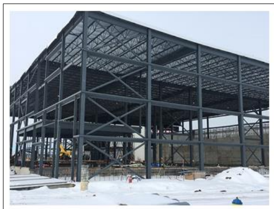
Figure 1.5: Multi-Tiered Braced Frame.
