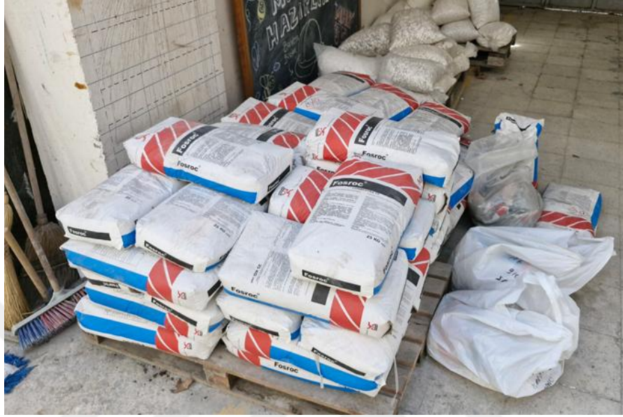
Figure 3.5: Storage of cement-based grout used in the mixture.
