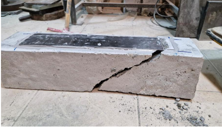
Figure 3.19: Deformation of the beams produced in the preliminary studies
