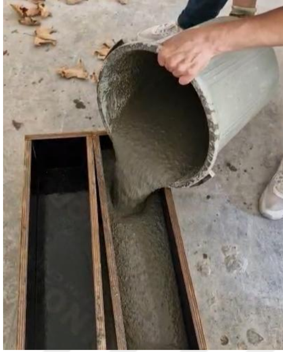
Figure 3.6: Placing the prepared mixture into molds.
