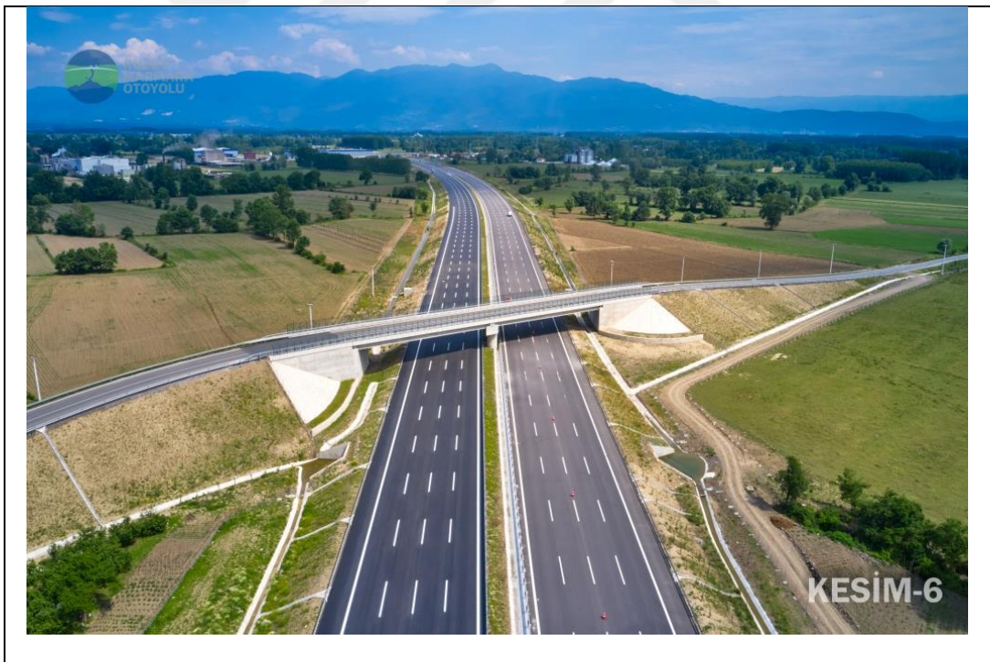
Figure 1.6: An overpass at the region 6 of the KMO.
