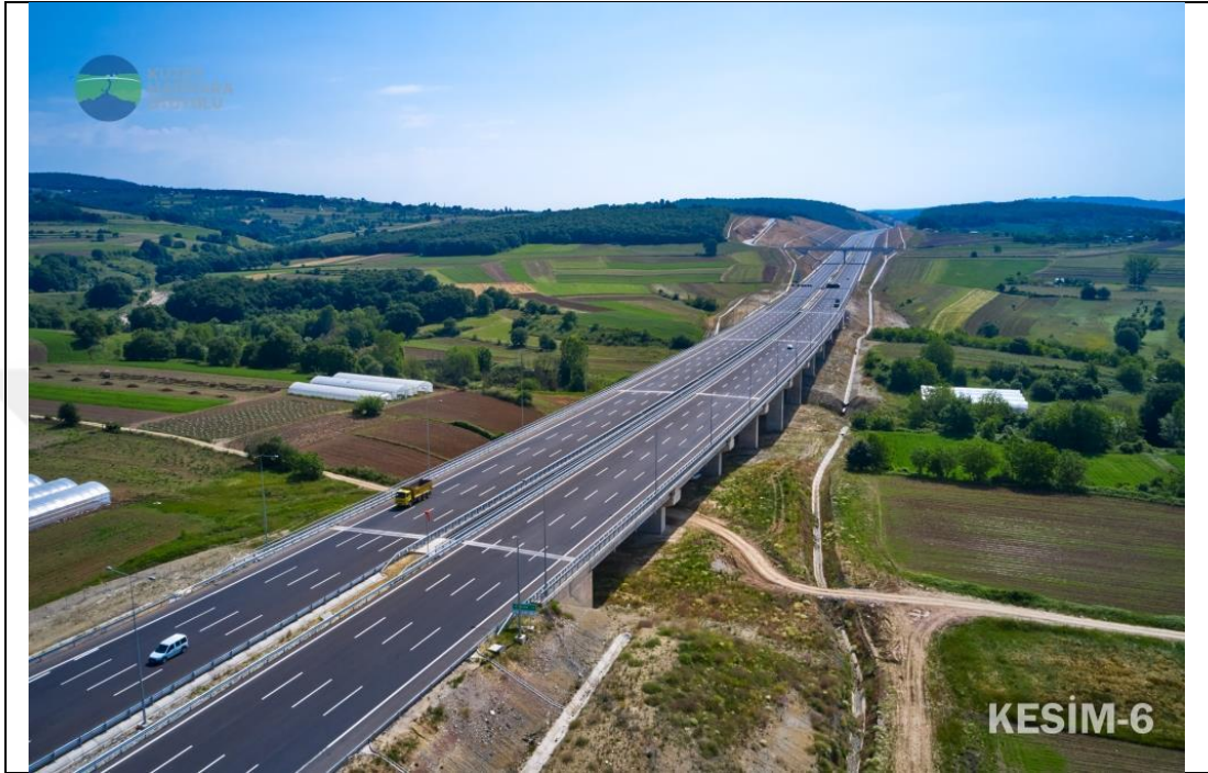
Figure 1.3: A viaduct at the region 6 of the KMO.
