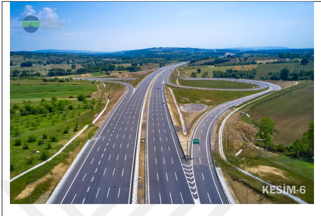
Figure 1.7: A partial cloverleaf interchange with an underpass and hydraulic culvert at the region 6 of the KMO.
