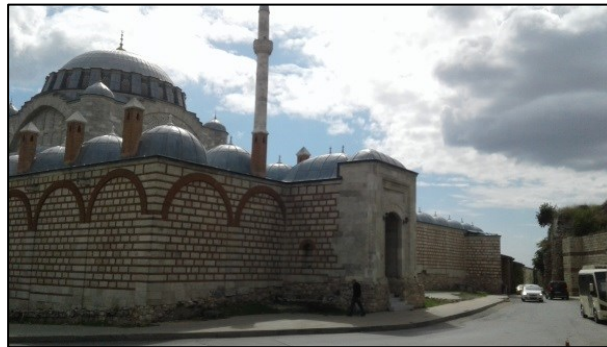
Şekil 3.42: E.M.M. yol cephesi (2017).
