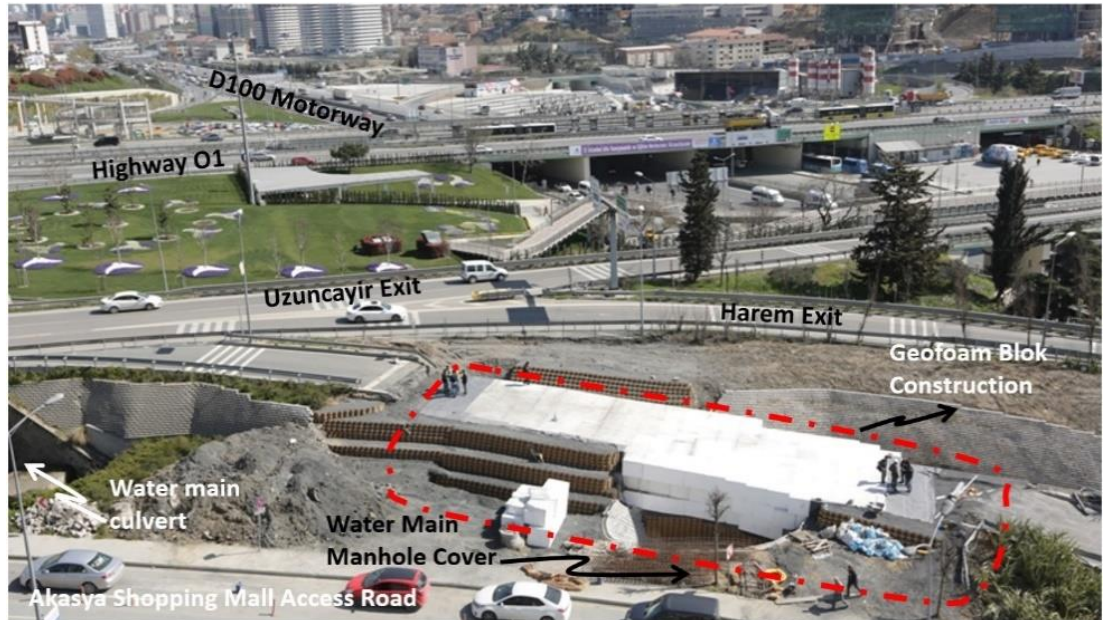
Figure 2.7: First Geofoam block road embankment project in Istanbul / Türkiye [Özer and Akınay, 2019].
