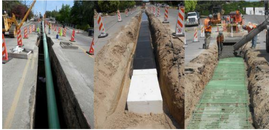
Figure 2.10: EPS Lightweight fill atop buried pipeline in Utah / USA [Bartlett et al., 2015].
