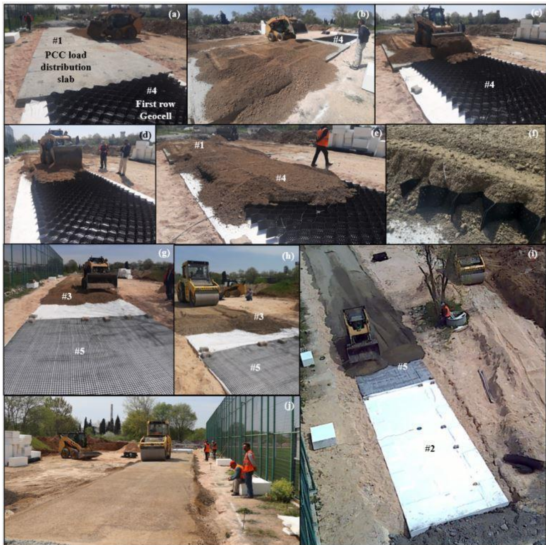
Figure 4.15: The first lift of granular base laying-compaction process, a-b) Placement of granular base atop the PCC slab in the Configuration #1 by pushing with a mini front-end loader, c-f) In-filling of geocell with granular base course at the Configuration #4, g-h) Laying of granular base at the Configuration #3, i) Laying of granular base at the Configuration #5, j) Compaction of loose granular base course material by a vibratory roller.
