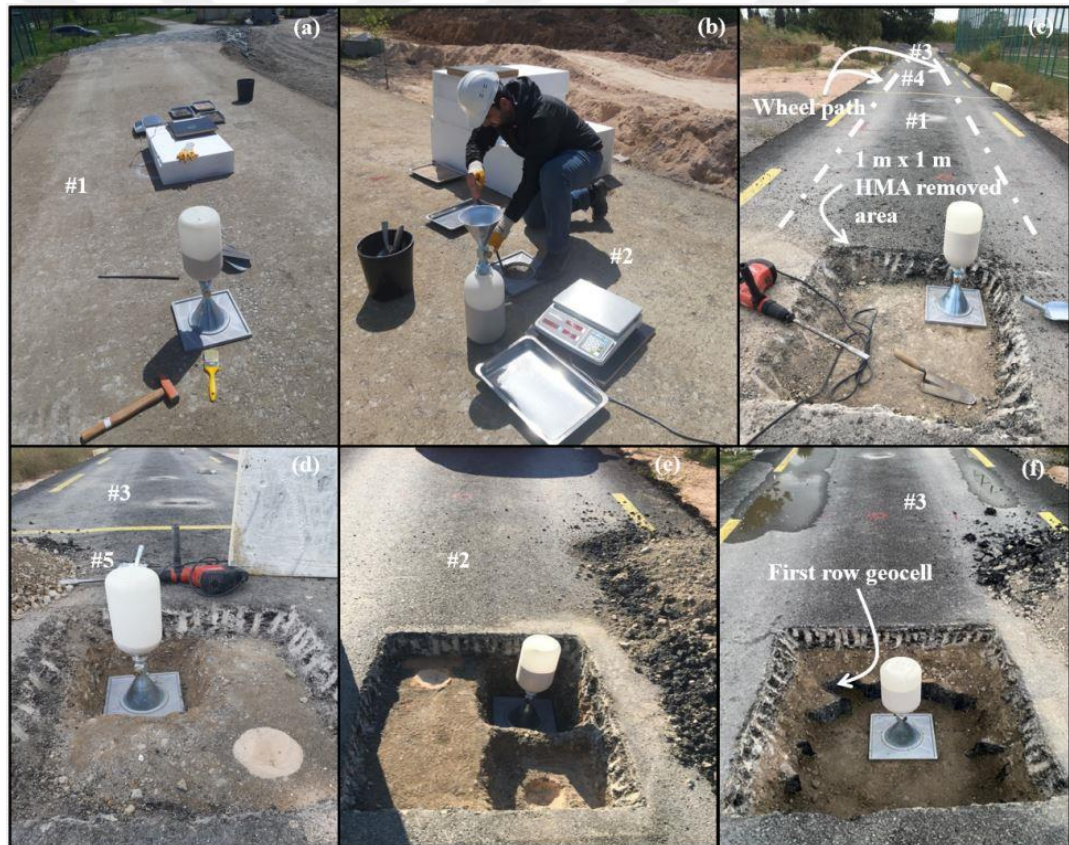
Figure 6.2: Sand cone tests, a-b) Prior to HMA construction Configuration #1 and #2, respectively, c-e) SC tests performed at different depths in Configuration #1, #5 and #2 upon completion of APT, f) SC tests performed beneath geocell at the Configuration #3.
