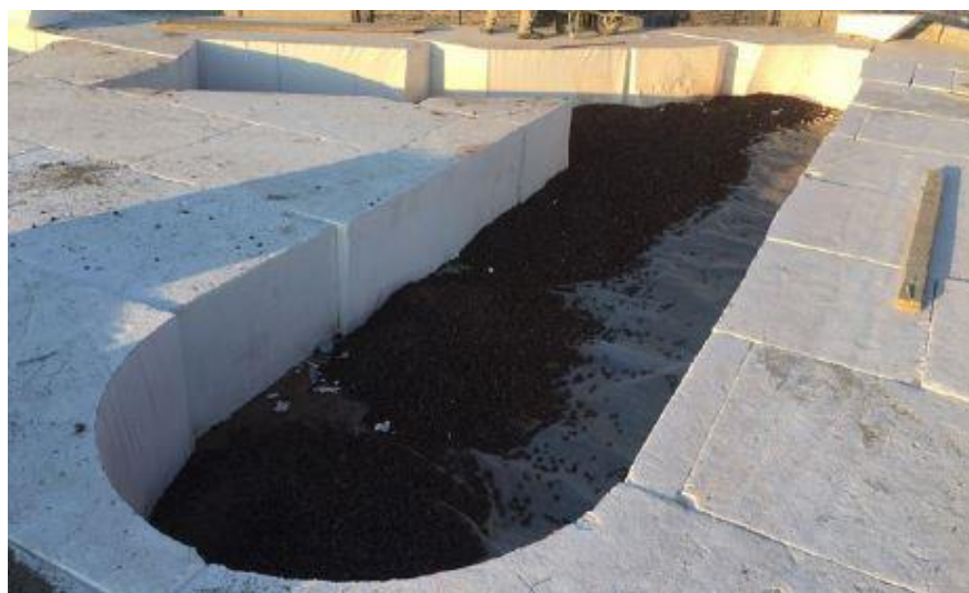
Figure 2.12: Geofoam block green roof application in Cesme / Türkiye [Özer, 2020].
