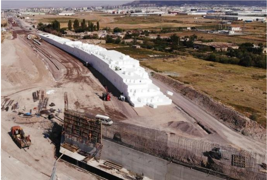
Figure 2.8: Geofoam block bridge approach road embankment in Kayseri / Türkiye [Özer 2021].
