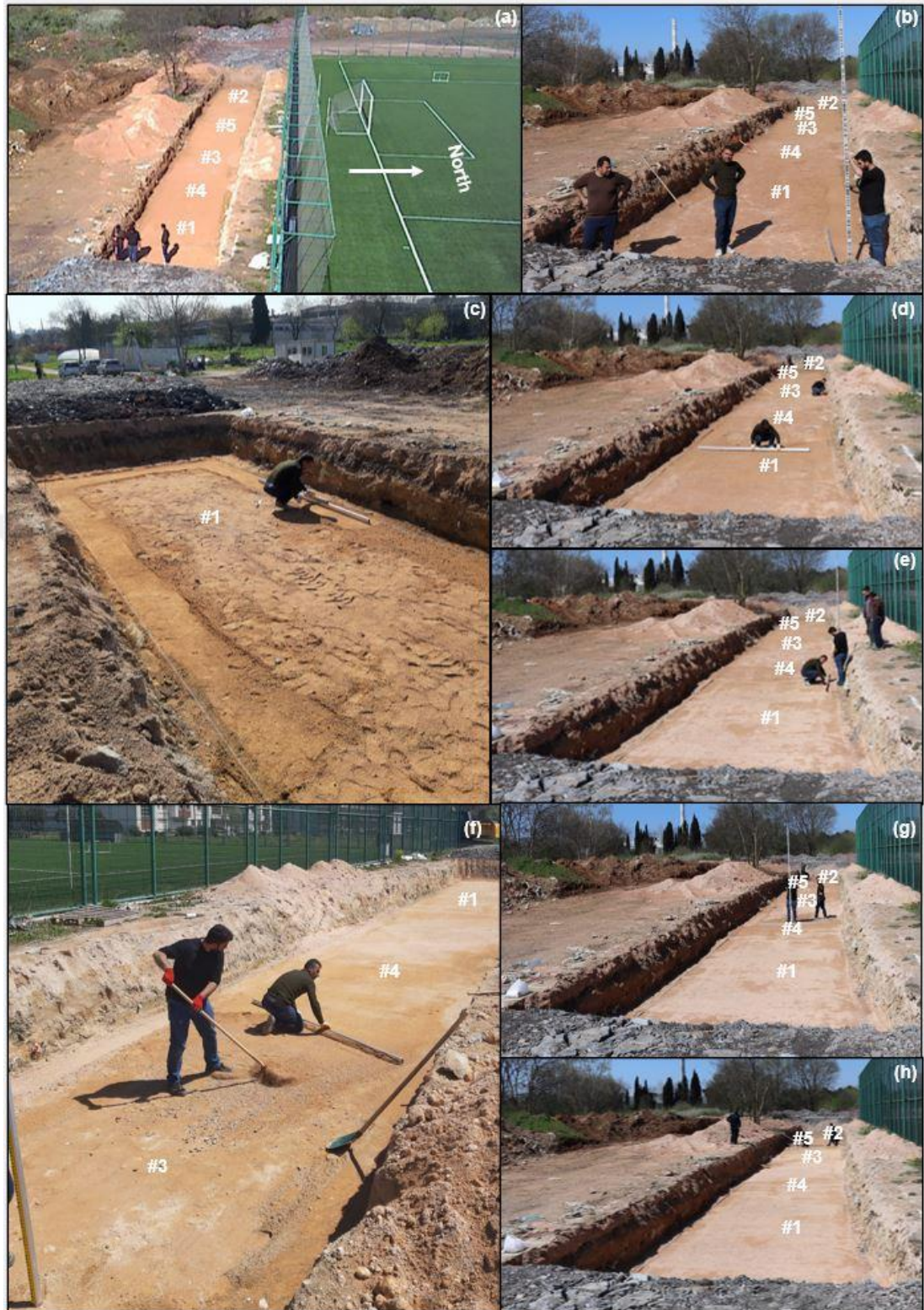
Figure 4.7: Final surface levelling with a aluminum straightedge (a) Completion of bedding sand laying, (b) Elevation control of the bedding sand layer before the start of the leveling, c-j) Completion of the bedding sand placement per project tolerance.
