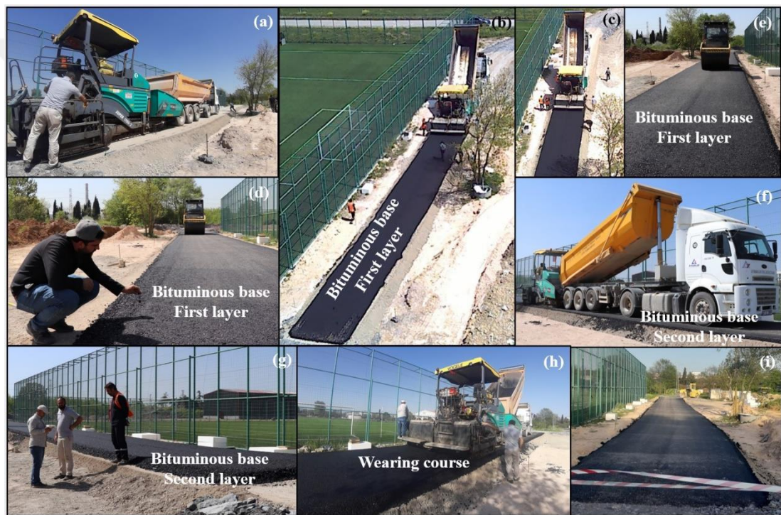
Figure 4.17: HMA laying-compaction process, a-c) Laying of first lift of the bituminous base, d) Temperature control prior to compaction, e) Compaction of first lift of the bituminous layer, f-g) Second lift of the bituminous base laying by a roadway finisher, h) Laying of wearing course layer, i) Completion of the HMA construction.
