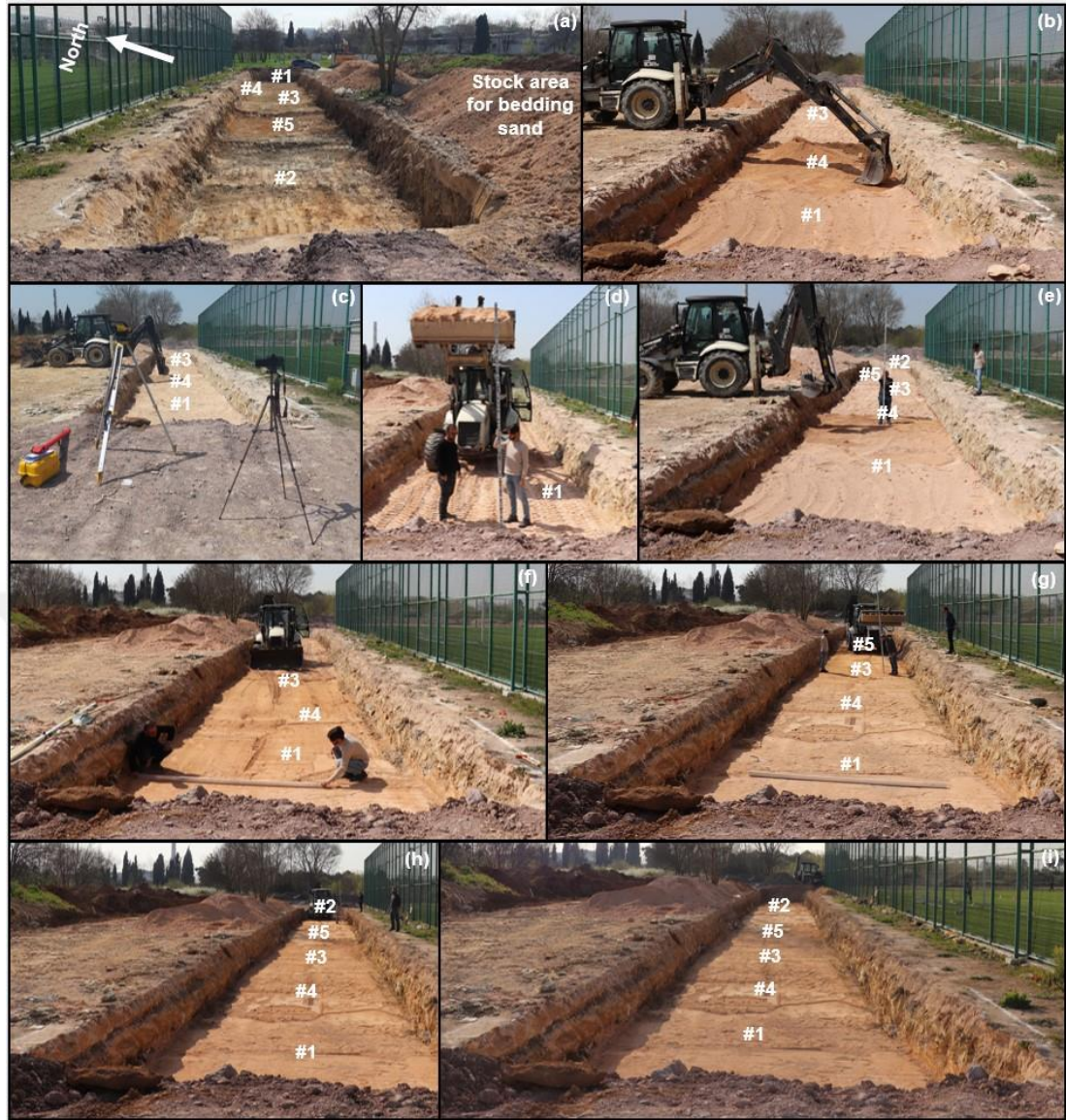
Figure 4.6: Bedding sand delivery, stockpiling and placement a) Transported bedding sand stockpiled at the west of the test bed excavation, b) Laying of bedding sand for Configuration #1, #4 and #3 with a wheeled backhoe-loader, c) Setting up of total station for elevation control of bedding sand, d) Elevation control in Configuration #1, e) Elevation control in Configuration #4, f-g-h) Laying of bedding sand with a wheeled backhoe-loader in Configuration #4, #5 and #2, respectively, j) Completion of bedding sand placement.
