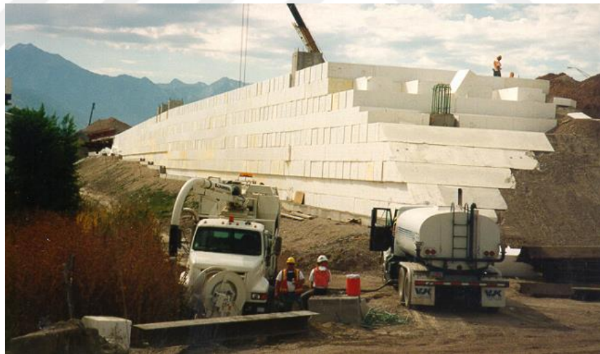
Figure 2.6: Geofoam block embankment in Highway I-15, Salt Lake City/USA [Newman et al., 2010].
