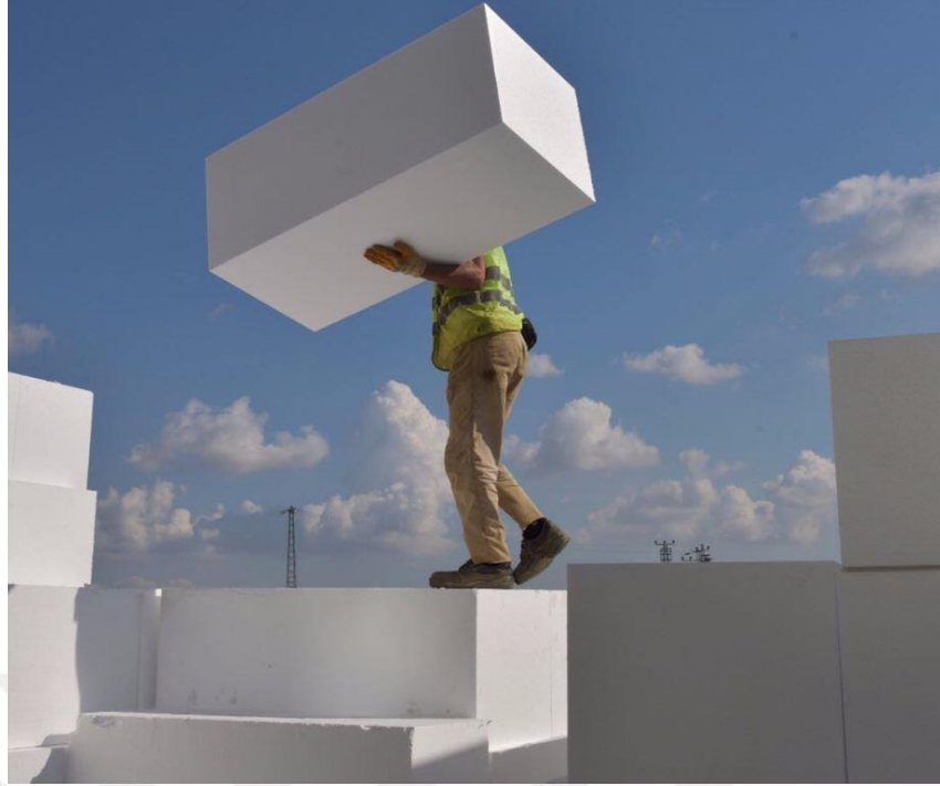
Figure 2.2: Geofoam block handling on-site [Özer, 2021].
