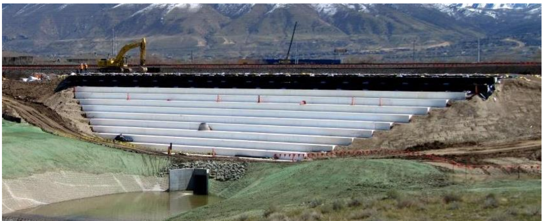
Figure 2.9: Geofoam block embankment constructed atop a hydraulic culvert in Utah / USA [Bartlett et al., 2015].
