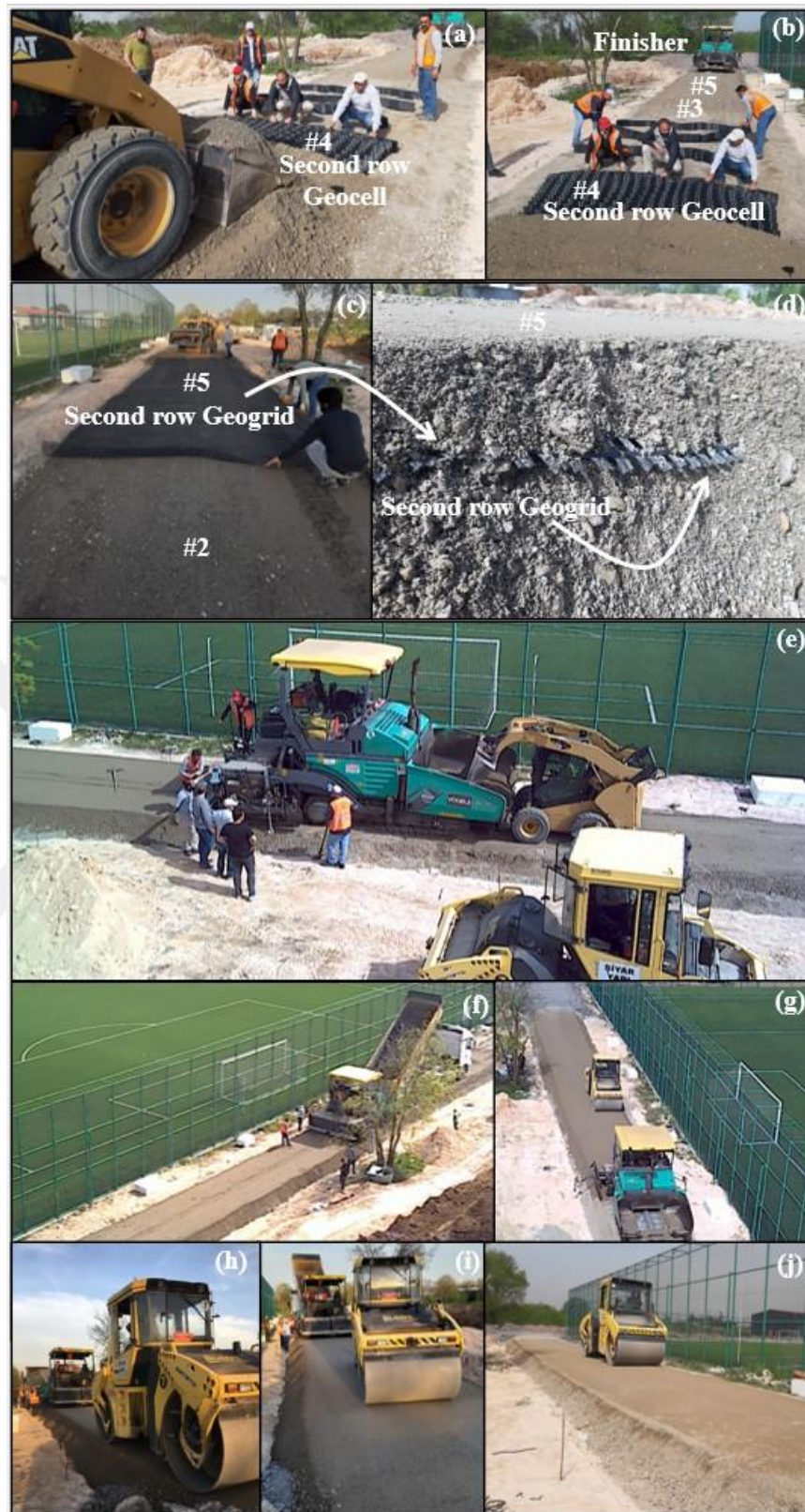
Figure 4.16: Second lift of the granular base laying-compaction process, a-b) Second row geocell placement at Configuration #4 and granular base laying, c- d) Second row geogrid placement at Configuration #5 and granular base laying, e-g) Second layer granular base laying by finisher, h-j) Compaction of granular base layer.
