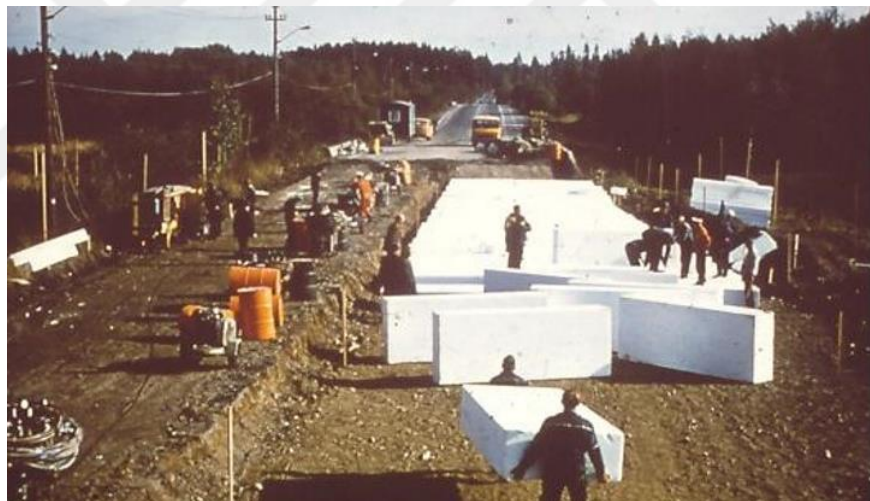
Figure 2.5: The first geofoam block embankment project – 1972, Norway [Aabøe and Frydenlund, 2011].
