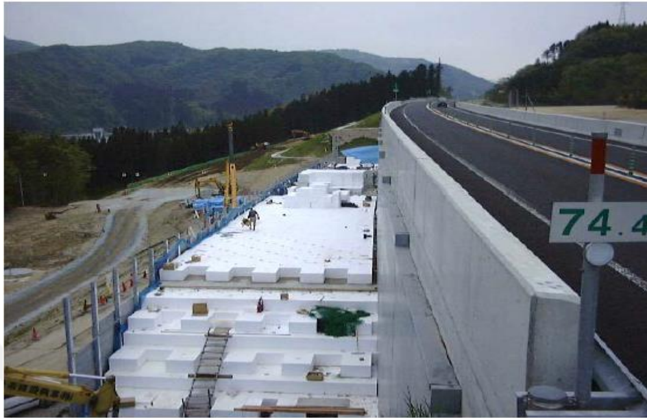
Figure 2.2: Using geofoam blocks in roadway widening application, Japan [Kawashima et al. 2001].
