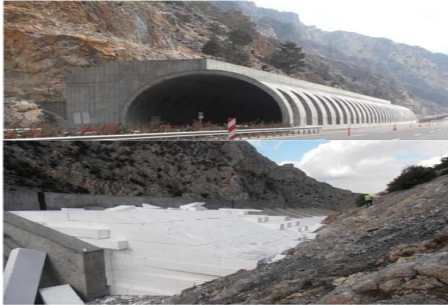
Figure 2.18: Geofoam blocks applied for energy absorption on rock fall protection tunnel in Turkey (Courtesy of EPSDER, Turkey) [Özer, 2020].
