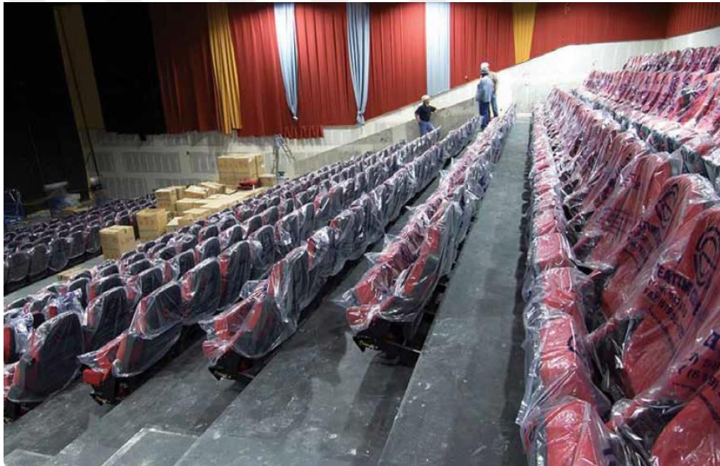
Figure 2.15: Stair-step geofoam block placement for seating arrangements [Stark et al., 2012].
