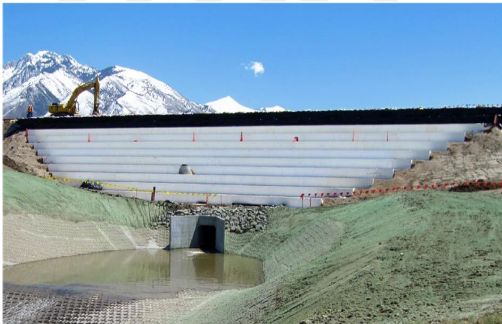
Figure 3.2: EPS geofoam embankment constructed over culvert system, Utah Transit Authority Frontrunner Commuter Rail System, Draper, Utah (photo courtesy of ACH Foam, Murray, Utah) [ Bartlett et al., 2015 ].
