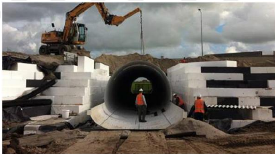
Figure 2.3: Construction of embankment around corrugated steel tunnel [Aaboe et al., 2019].
