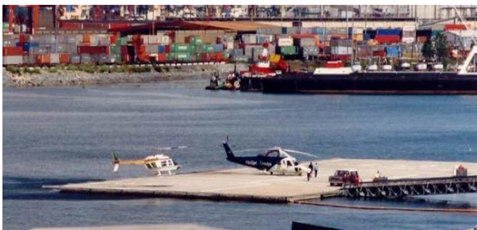
Figure 2.19: Floating helipad supported by geofoam blocks (Vancouver, Canada) [Aabøe et al., 2012].
