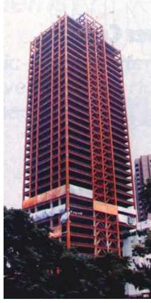
Şekil 2.6: Tuntex Construction Company (39), Taipei, Tayvan.
