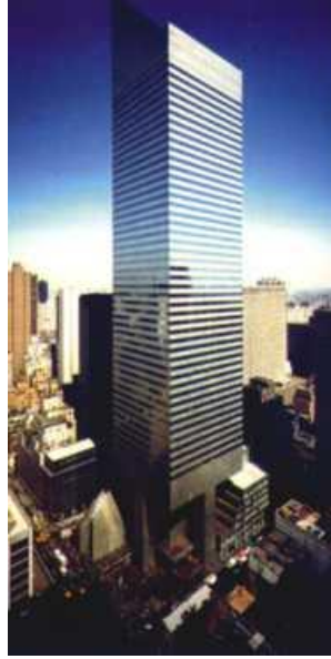
Şekil 2.5: Citicorp Center (278.6 m - Tuned Mass Damping System) - New York.
